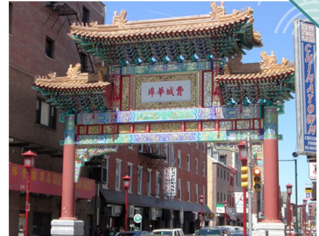
Figure: gate of Chinatown on 10th St (Source: Wikipedia)
