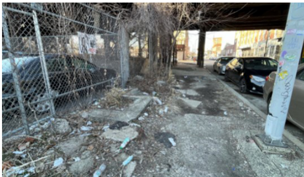
Figure: the 10th St Park and wasteland land under The Rail Park. (Source: Authors, 2022)
