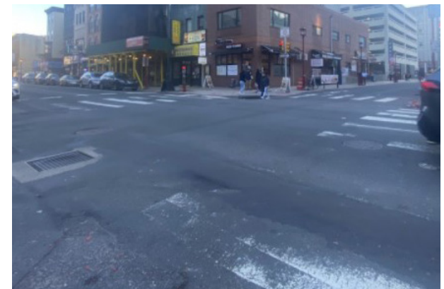
Figure: Example of faded crossings: The entrance of Chinatown on 10th Street (Source: Authors, 2022)
